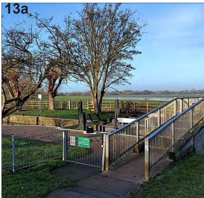
13a: Lock and bridge over Great River Ouse
