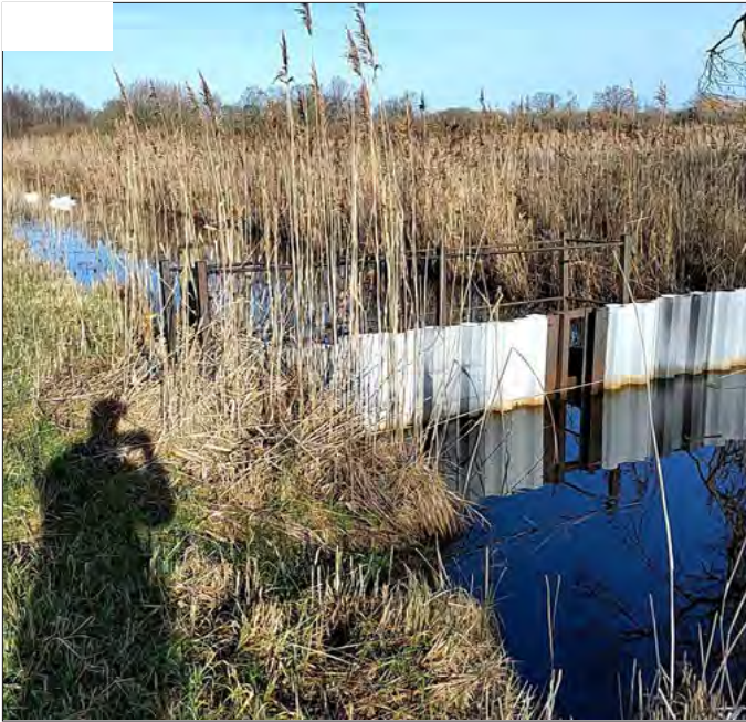
23: Management of watercourses on site
