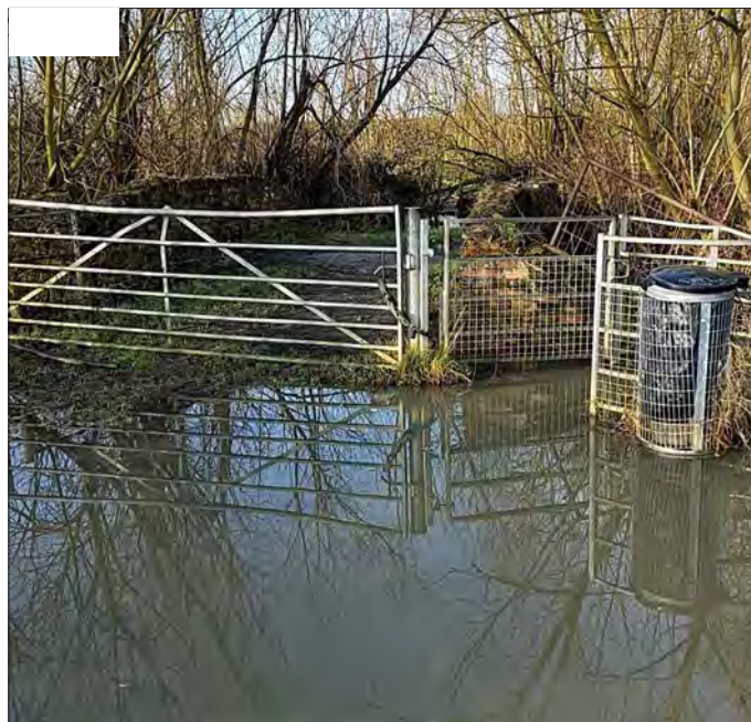
22a: Flooded entrance to Portholme
