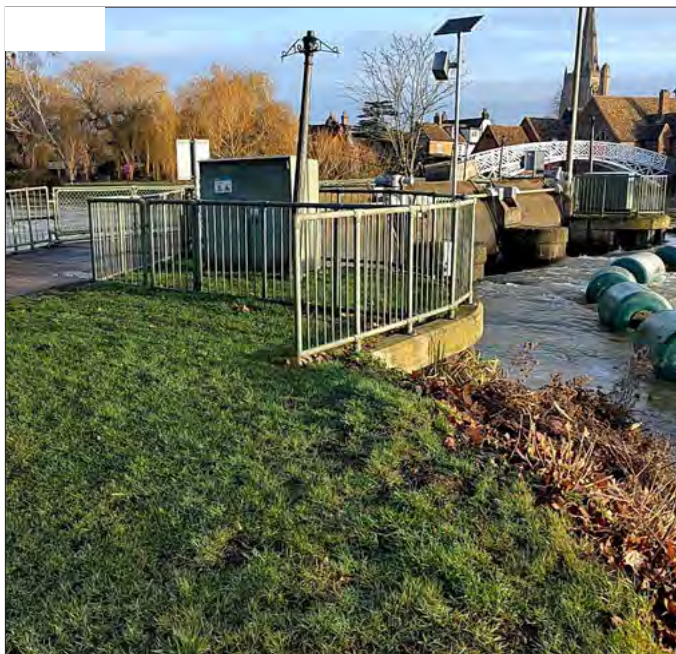
5: Bridge and sluice over Great River Ouse
