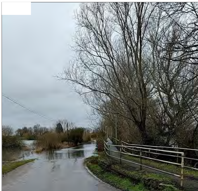
25b: Flooded road access and pedestrian walkway
