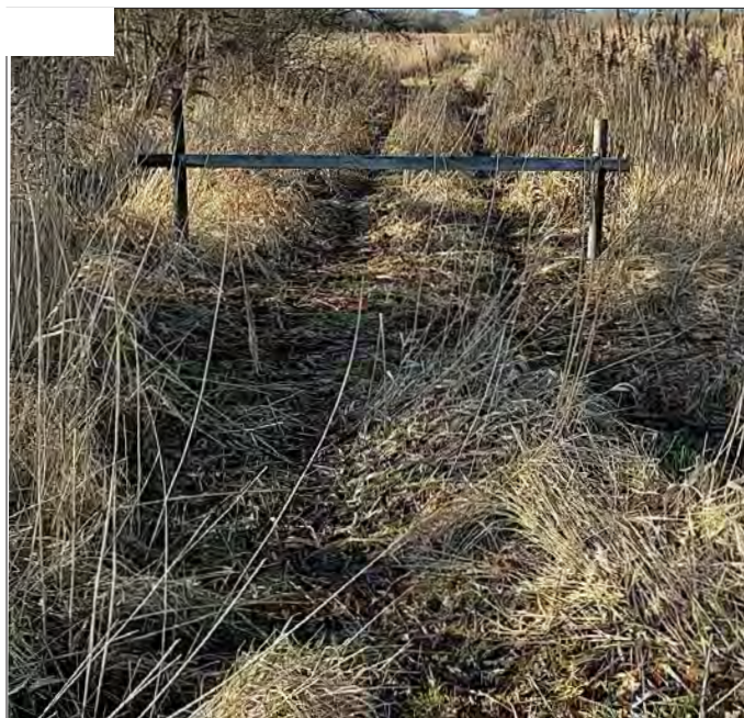
20: Blocked access to sensitive area of site
