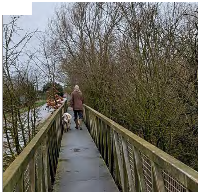
29: Dog walker utilising raised pedestrian walkway
