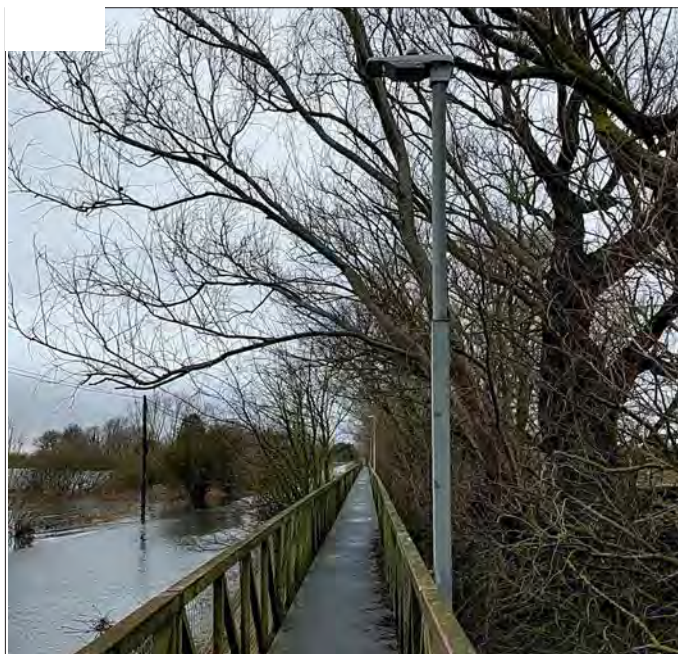
25c: Pedestrian raised walkway and lighting
