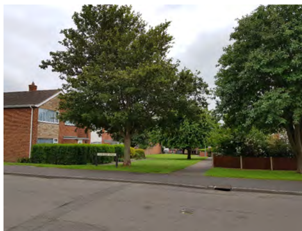
Ashbridge Walk is one example of properties facing onto amenity space
