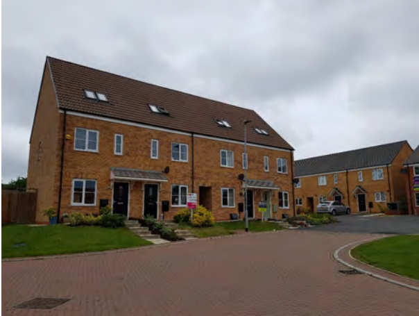
Terraces within Whitney Drive overlooking a central green space and areas of parking
