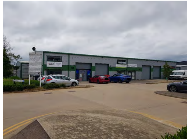
Enterprise Court within the Eagle Business Park
