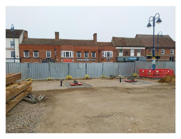
07/05/2024 – Completed rain garden system installation after backfilling. Holes covered in preparation for tree planting.
